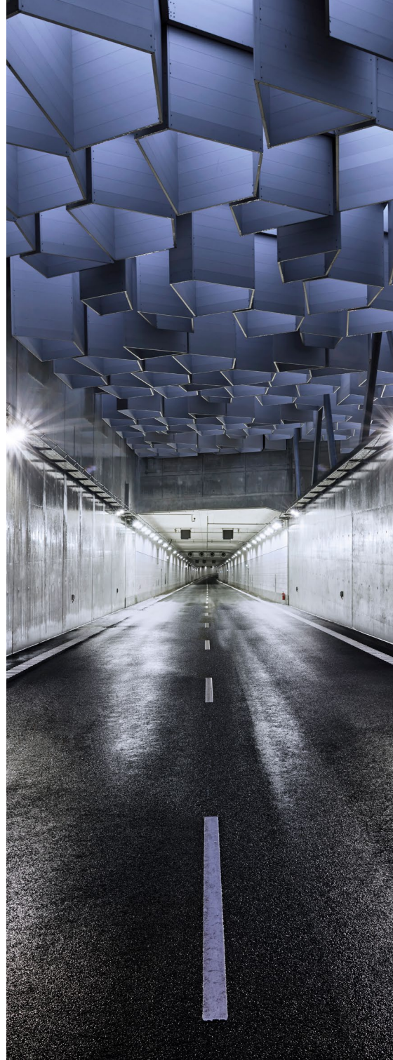
Nordhavn Tunnel Denmark
